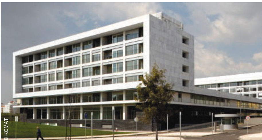
Hospital da Luz, Lisbon - Portugal
